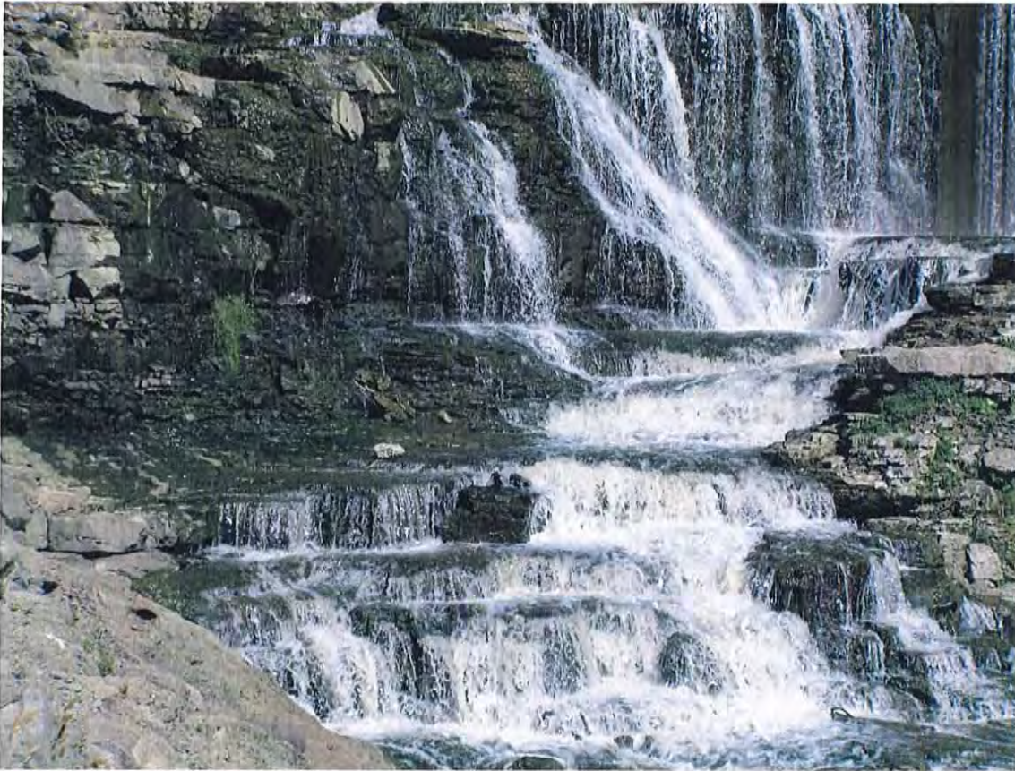
Side Spillway of the O'Shaughnessy Dam Scioto River Watershed
