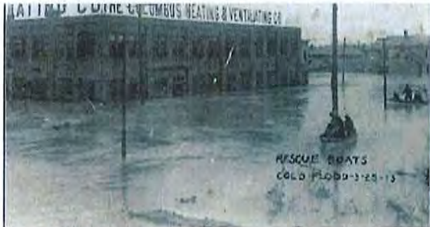
1913 Flood: Hundreds killed and thousands of buildings damaged in Columbus www.dispatch.com
