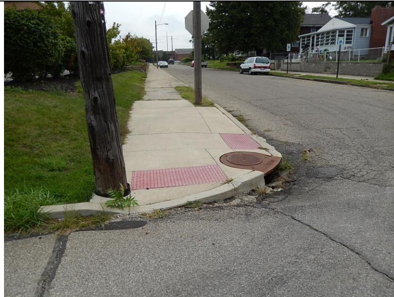
ADA ramp at Lexington and 3 rd –may be difficult to use due to large curb.
