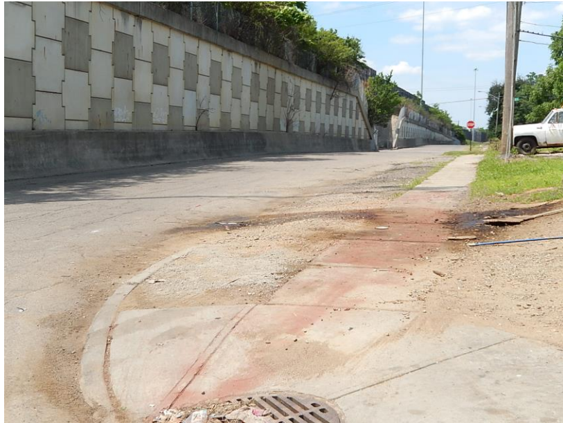
Howard- debris present with deteriorating buffer. Also note overgrowth of trees on retaining wall-hazardous to walkers.
