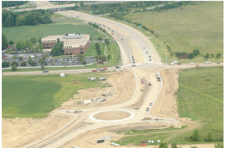
Aerial photograph of construction in progress of a new round-about for the N. Hamilton Road “S” curve at State Route 161.
