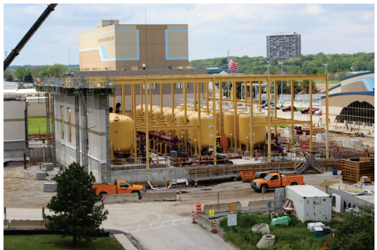
Construction on the new ion exchange treatment portion of the DRWP Capacity Increase.
