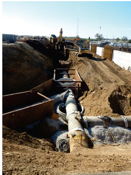
Installation of a new clearwell at PAWP. This will increase the reliability of the water supply system.
