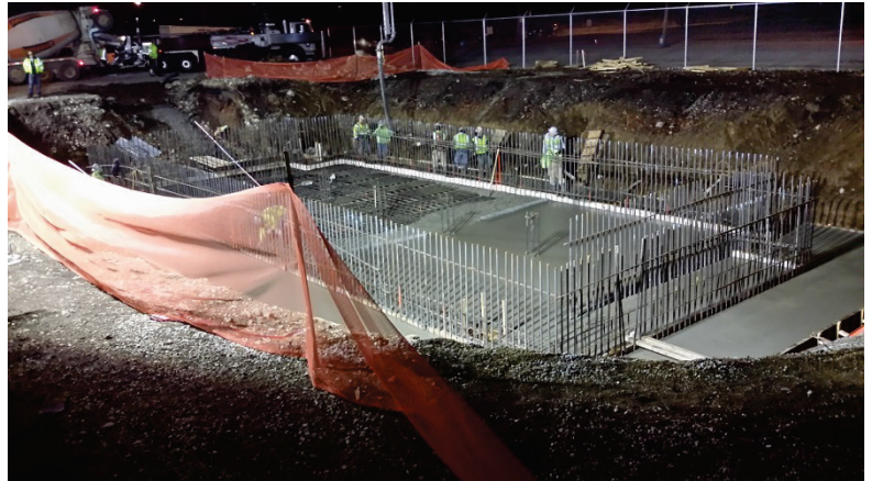
Crews work through the night to install the new foundation for the Dublin Avenue Substation.
