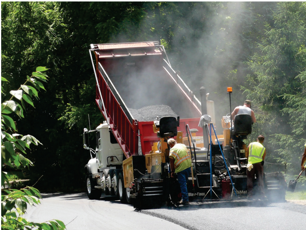
Road being resurfaced with new asphalt as a continued part of the city's resurfacing commitment.
