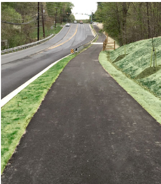
Shared Use Path – New 10' wide asphalt path along corridor for pedestrian and bicyclists
