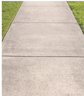
Concrete Sidewalk – New 5' wide concrete path along corridor for pedestrians
