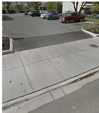
Drive Apron – New drive aprons and curb cuts along corridor for more defined vehicle access
