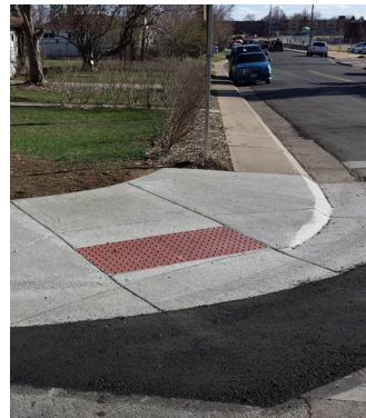
Curb Ramps – New curb ramps to meet ADA standards
