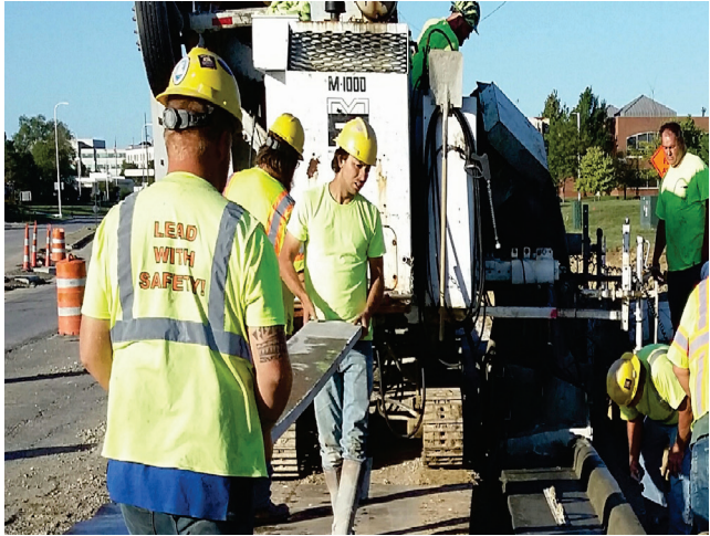
Curb Installation on Polaris Parkway
