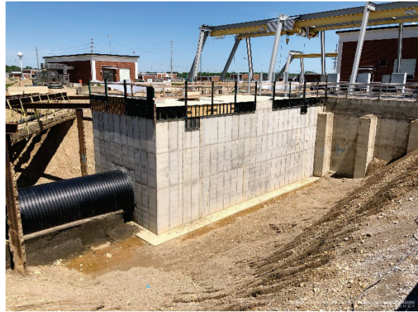
Photograph of the construction of the CEPT Dechlorination Structure at the Southerly Wastewater Treatment Plant.
