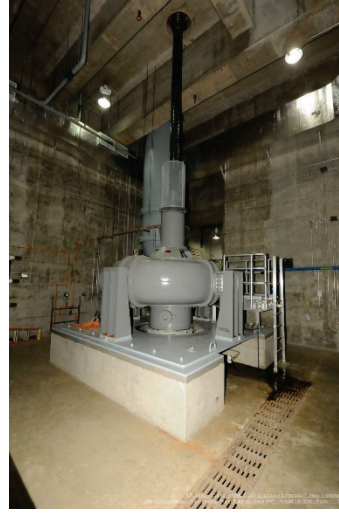
Photograph of a new Raw Water Sewage Pump at the Southerly Wastewater Treatment Plant.
