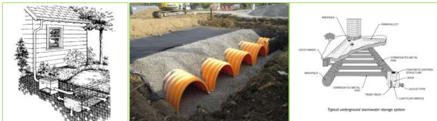
FIGURE 4-5 TYPICAL UNDERGROUND STORAGE CHAMBER CONFIGURATIONS
