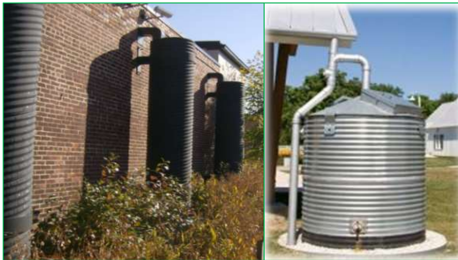
FIGURE 4-4 TYPICAL ABOVE-GROUND RAINWATER HARVESTING CISTERNS
