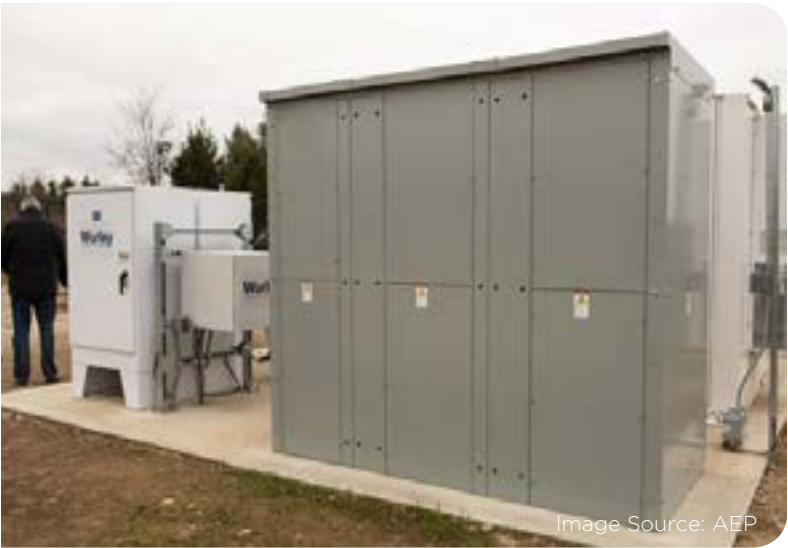
A 1,200 kWh battery energy storage system at the Columbus Zoo serves the critical saltwater life support for the polar bear exhibit.
