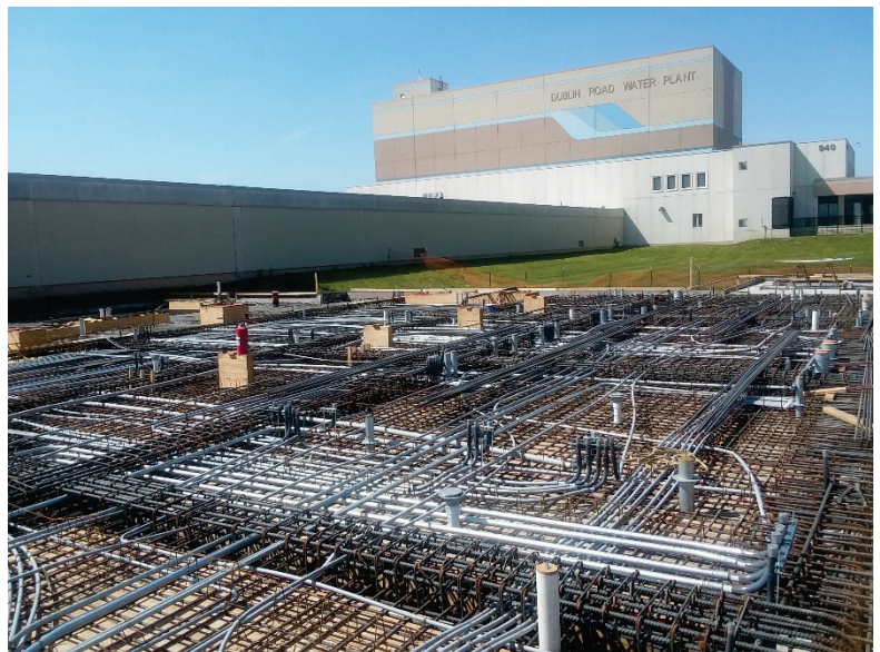
Installation of rebar and conduit in the DRWP UV Facility's first floor slab
