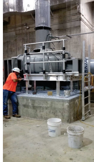
Installation of the Access Platform for RSP 1 at the Southerly Wastewater Treatment Plant.
