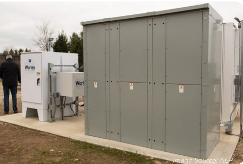
A 1,200 kWh battery energy storage system at the Columbus Zoo serves the critical saltwater life support for the polar bear exhibit.
