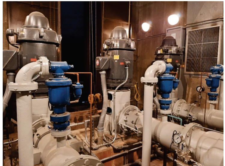
View of the PAWP CW104 new motors for the three vertical turbine pumps
