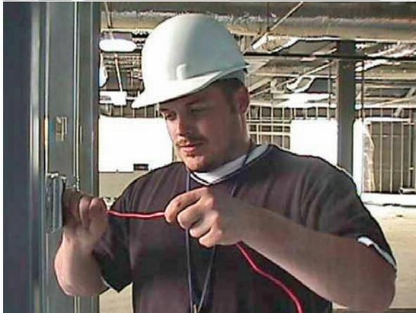
A. At the stage the contractor has installed the alarm device boxes and wiring in the rough walls (e.g. pull stations, horns, strobes, etc.) it will be necessary that these installations be inspected by the Electrical Inspector.
