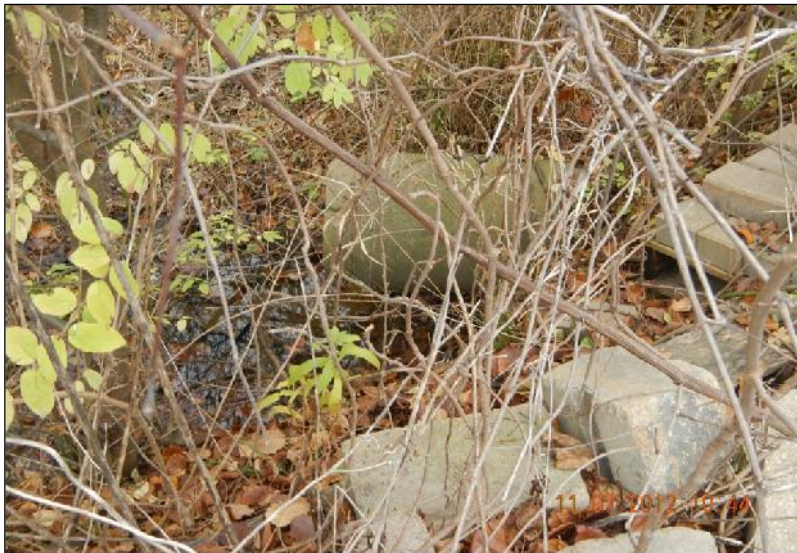
Photo 7 – Photo showing 12 inch culvert on the North bank of Stream 1A . Stream 1A becomes intermittent from this point.
