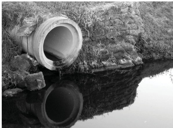
When water enters a stormwater inlet, it flows through underground pipes and empties directly into a nearby stream or river.
