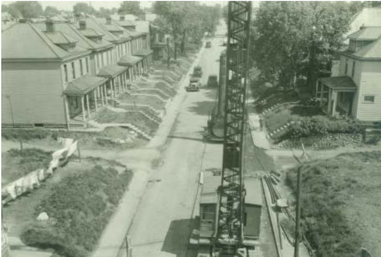
A street view of construction on Oregon Avenue sometime between 1931 and 1940.
