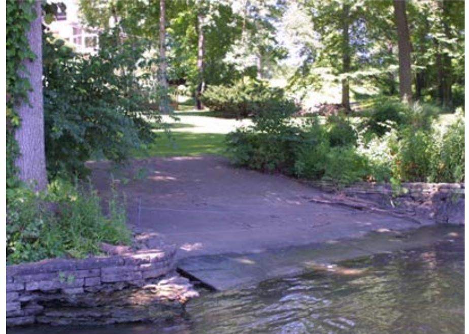
Unauthorized ramp allowing stormwater to flow directly into reservoir with no filtering.
