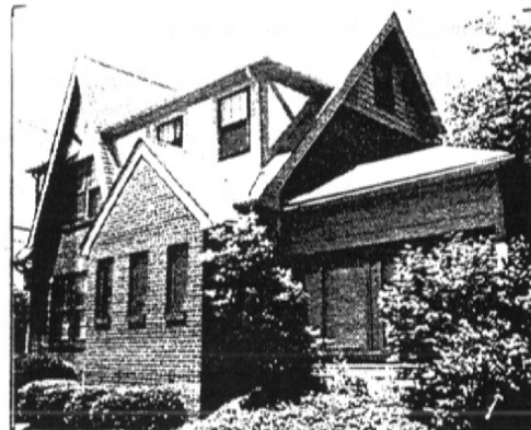
Residential building with dormer and addition.
