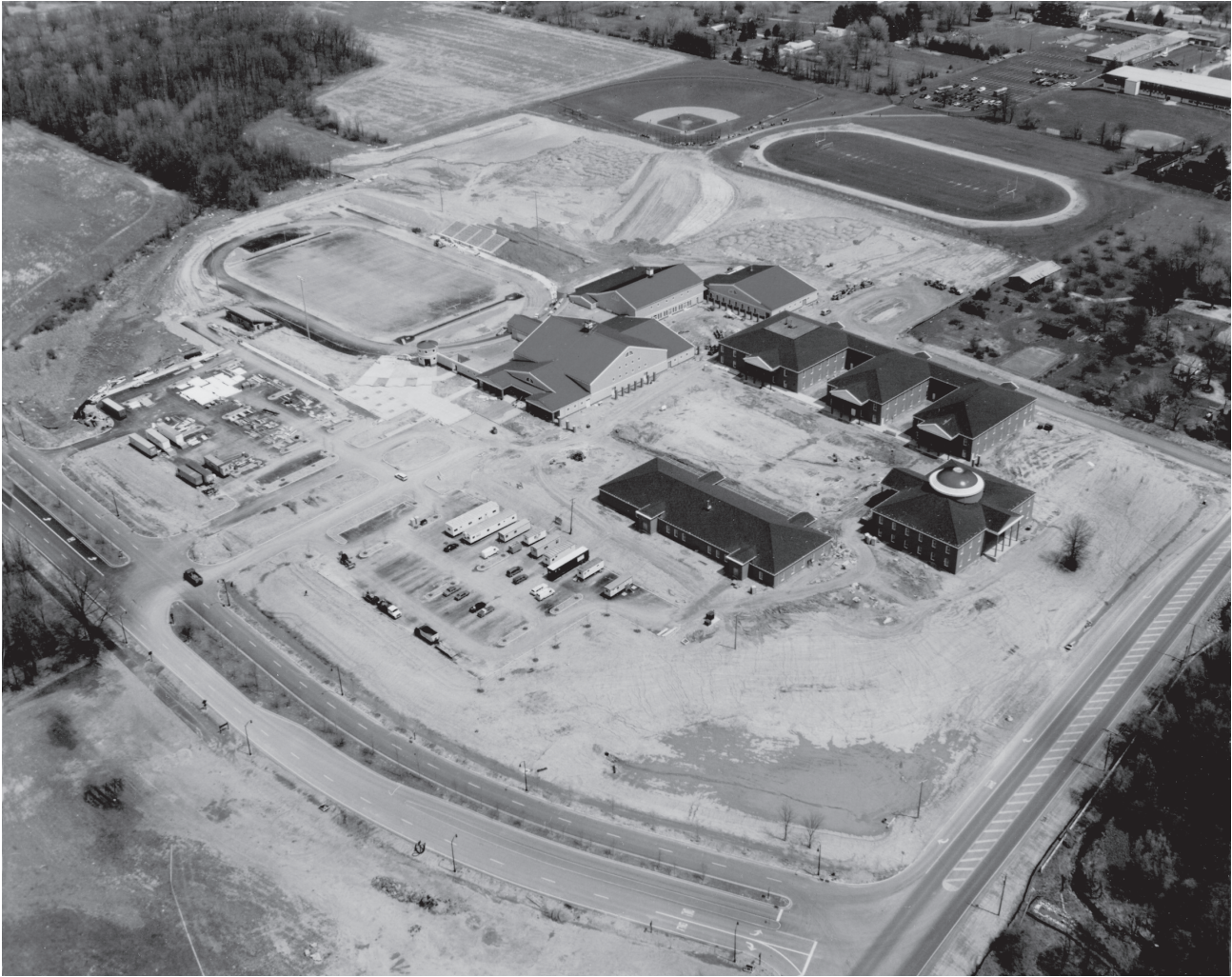
New Albany High School During Construction – June 1996
