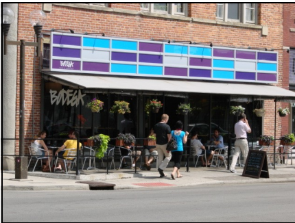
Canopies should enhance the entrance to a building, drawing visual design cues from the exterior design, materials and colors.
