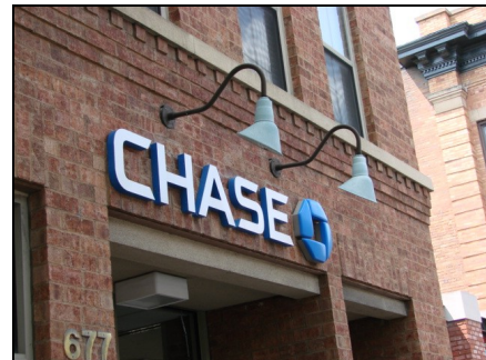
Goose neck fixtures illuminating a wall sign.
