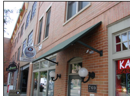
Awnings should be flat sloping with open ends, with supporting structures an integral part of the design and painted with low contrast colors.
