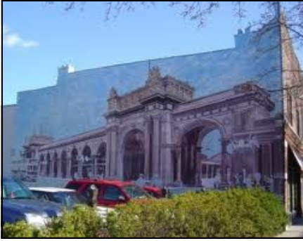
Murals are best located on “party” walls that existed between buildings. They can enhance the built environment, especially adjacent to surface parking lots.
