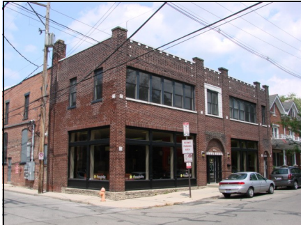
Examples of typical 20th century facades...
