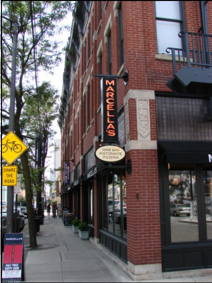
The Yukon Building is an example of a structure cited with a zero-foot setback off of the right-of-way of High Street.
