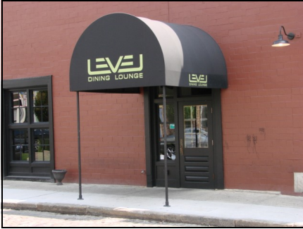
Awnings placed at a building entrance, perpendicular to the building elevation, are considered to be entrance canopies.
