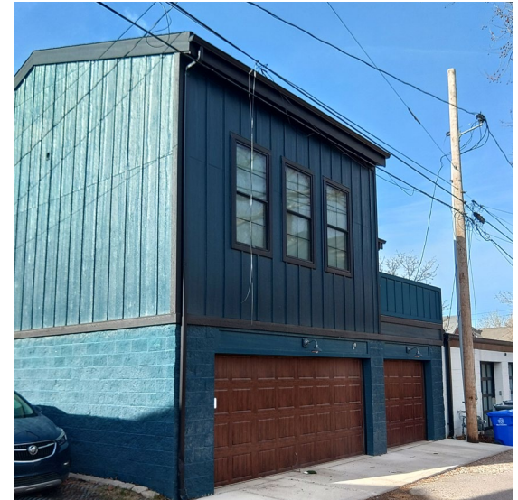
A detached, two-story ADU built above a garage.
