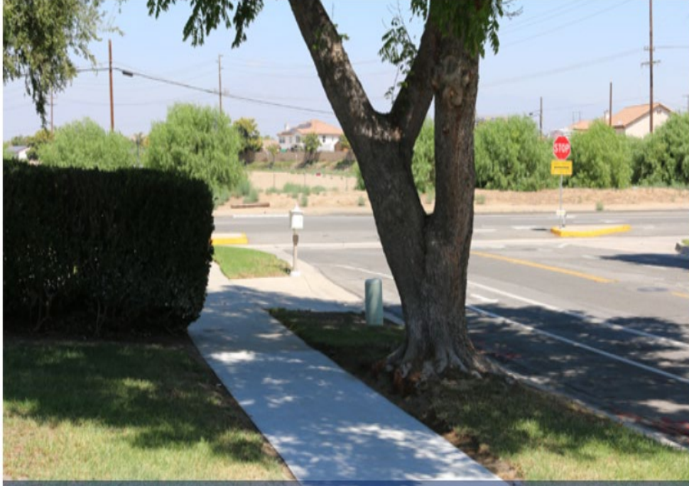
Figure G13. Rubber sidewalk near tree. Source: Rubberway (rubberway.com)
