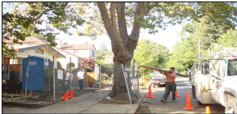
Figure 6: Tree protection fencing for a street tree in a tree well. Source: DeepRoot.com
