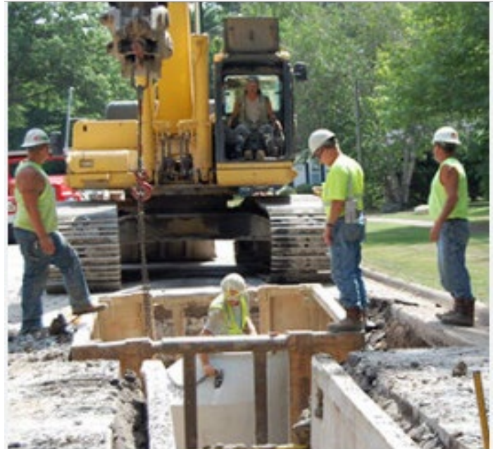
Installation of Sanitary Sewer
