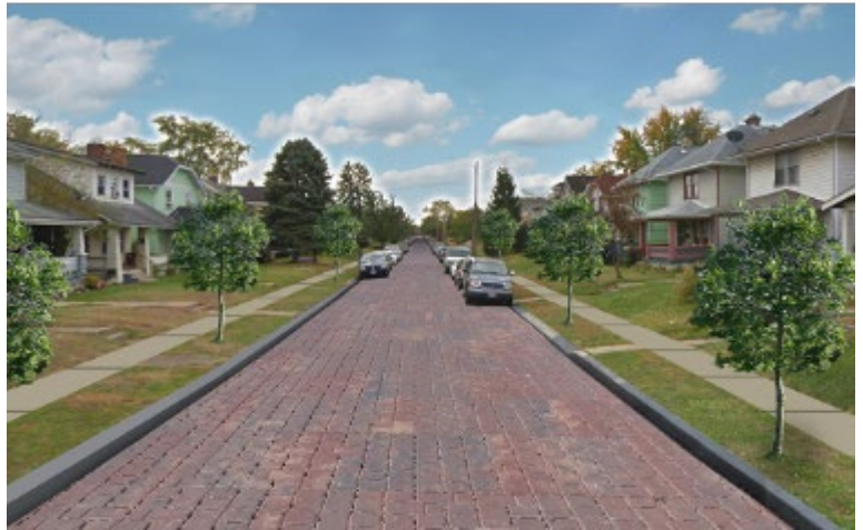
Permeable Pavers Installed on a Columbus Street
