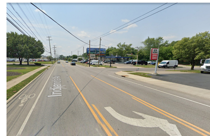
Parsons Ave Road Diet
