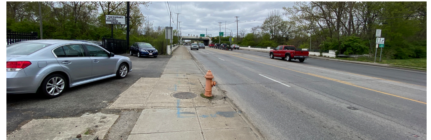
Unsafe pedestrian/sidewalk conditions
