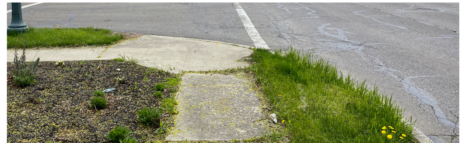
Unsafe pedestrian/sidewalk conditions
