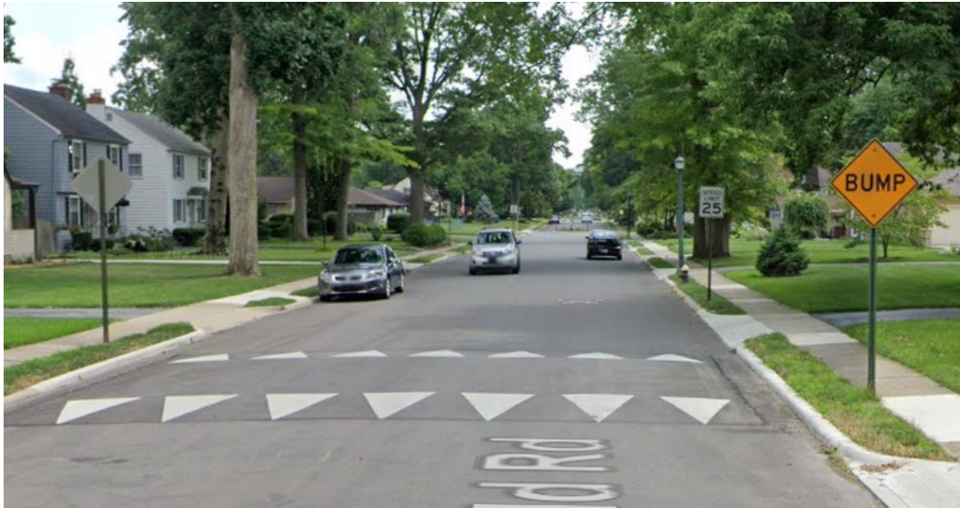
Figure 3. Example of Speed Hump on Nearby S Gould Rd
