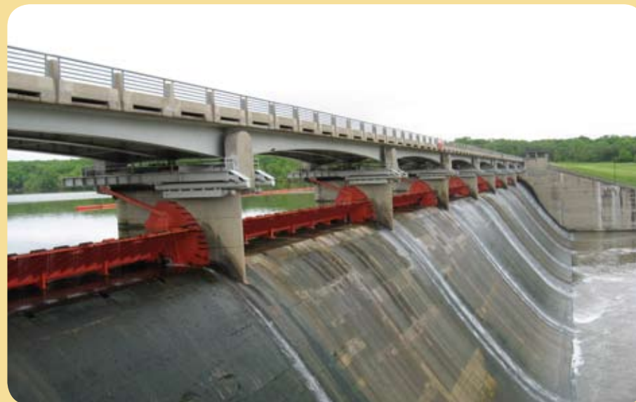
Hoover Reservoir Dam
