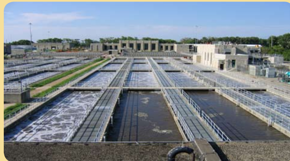
Jackson Pike Wastewater Treatment Plant
