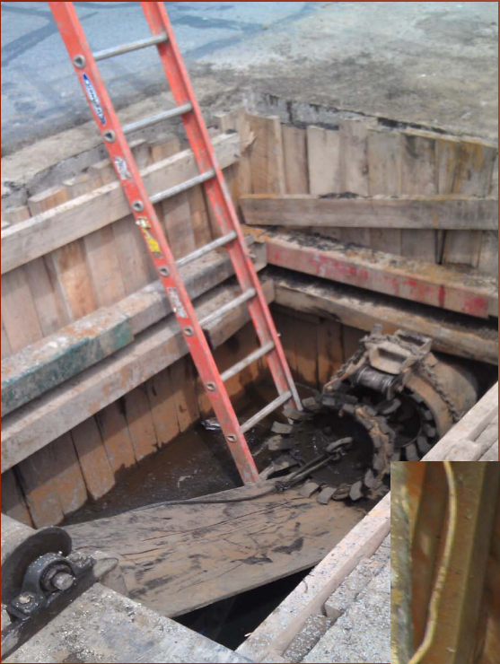
Sullivant Avenue Water Line Cleaning and Lining
