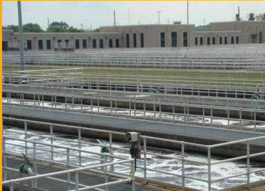
Jackson Pike Wastewater Treatment Plant
