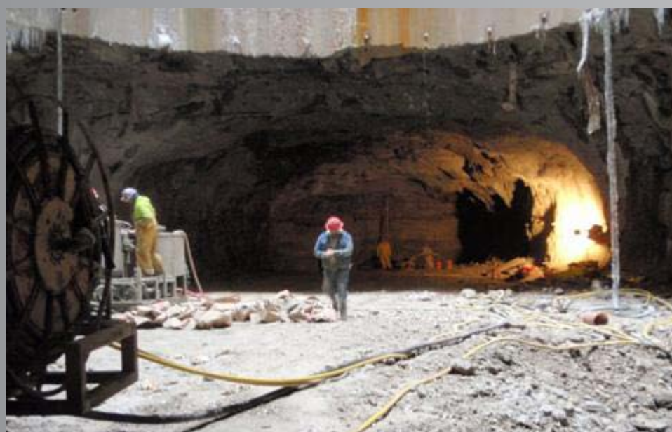
Tail Tunnel, OARS Phase 1
