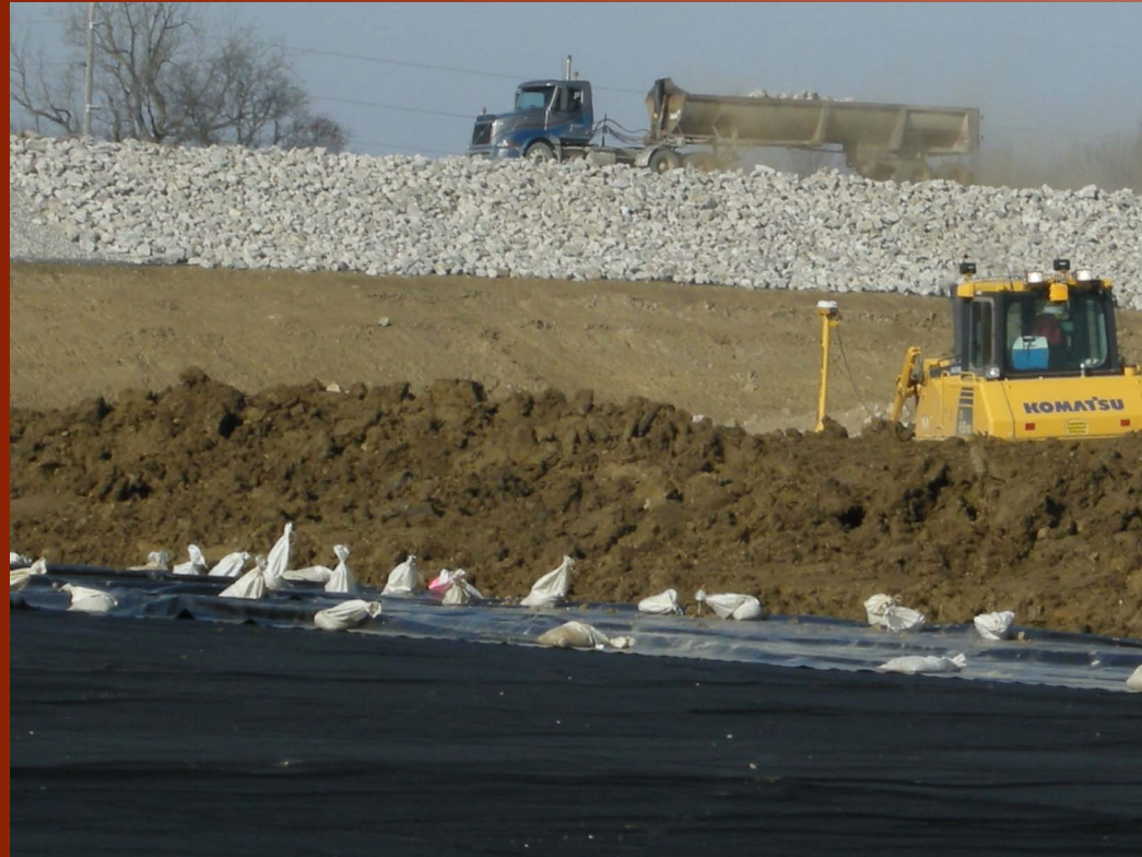
Construction at the Upground Reservoir
