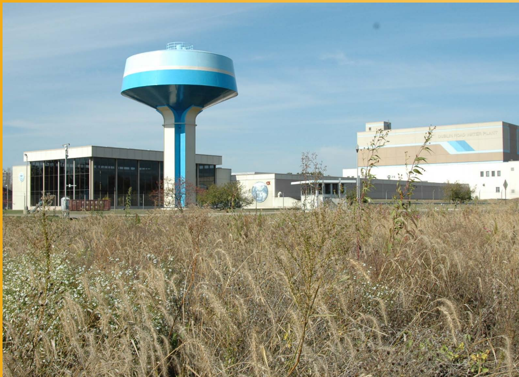
Dublin Road Water Treatment Plant
