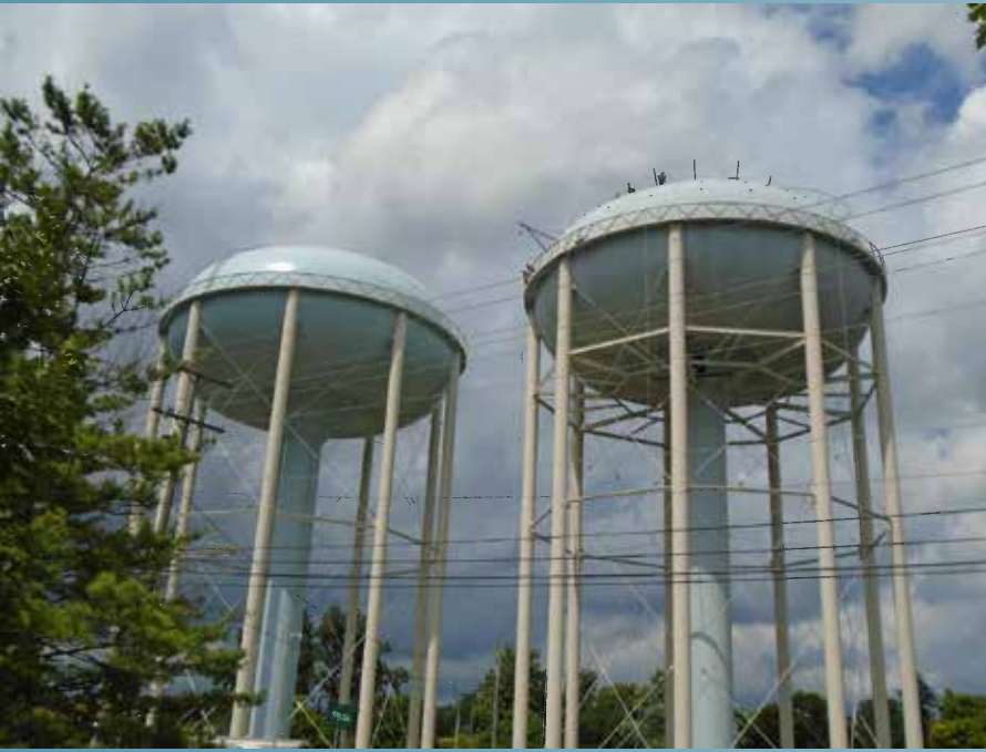
Henderson Road tank refurbishing underway
