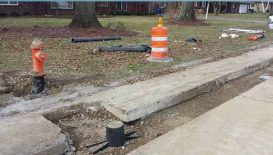
Cooke Road water line work
