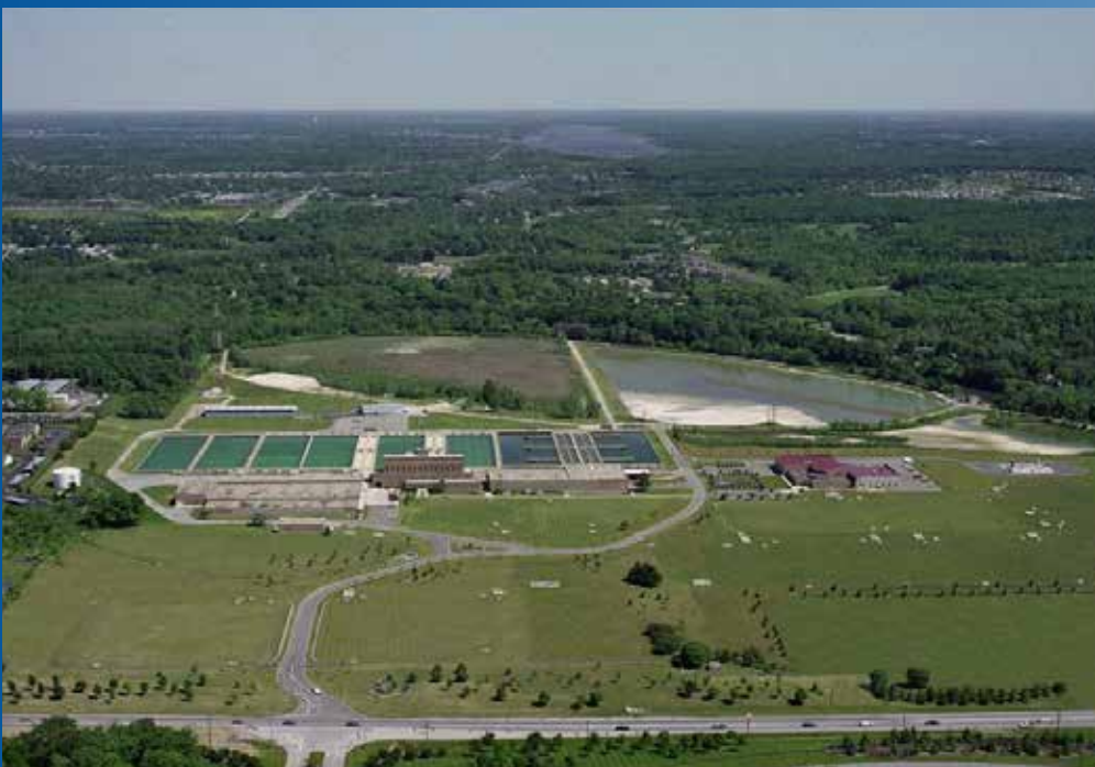
Hap Cremean Water Plant, with Hoover Reservoir visible to the north
