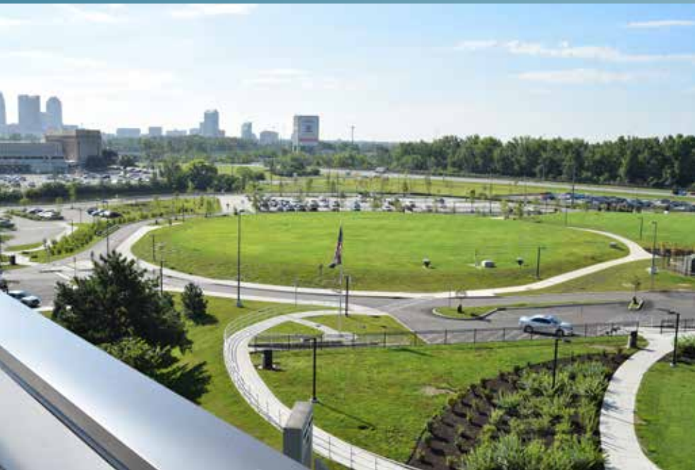
Relocated and expanded parking, sidewalks and green space at the Dana G. "Buck" Rinehart Public Utilities Complex at 910 Dublin Road
