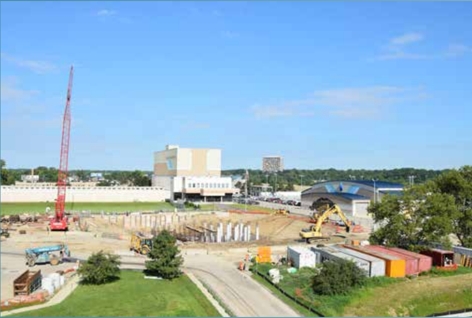
Dublin Road Water Plant treatment expansion under construction
