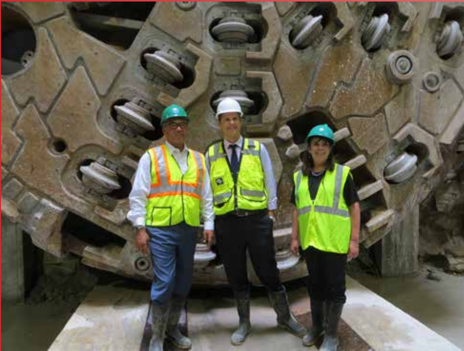
Mayor Michael B. Coleman and Councilmembers Zachary Klein and Eileen Paley in front of “Marsha,” the OARS tunneling machine after it bored through to the shaft at Neil Avenue and Vine Street, completing its journey
