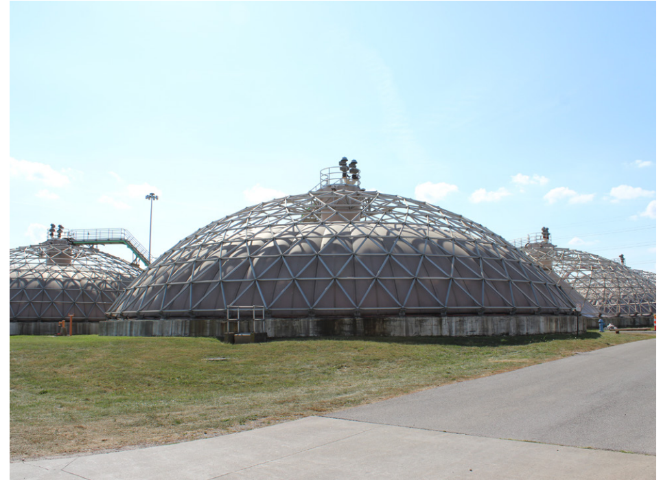
Sludge digesters at Jackson Pike WWTP, visible from I-71 south of downtown
