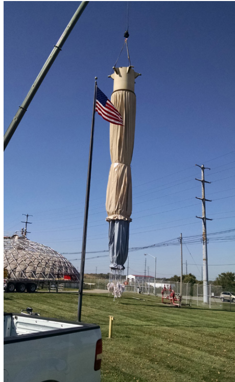
Jackson Pike Digester Cover Replacement
