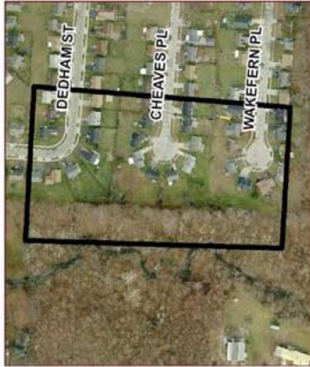
Figure 2. Framingham Circle: erosion at four existing storm sewer outfalls
