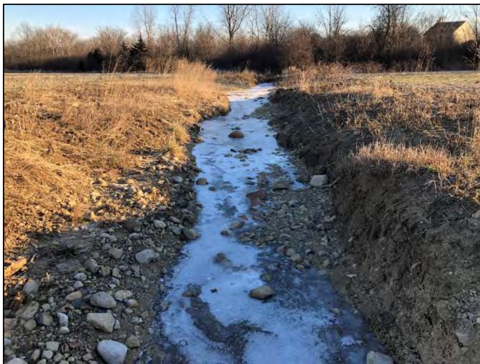
02 - Viewing ST-001 downstream.
