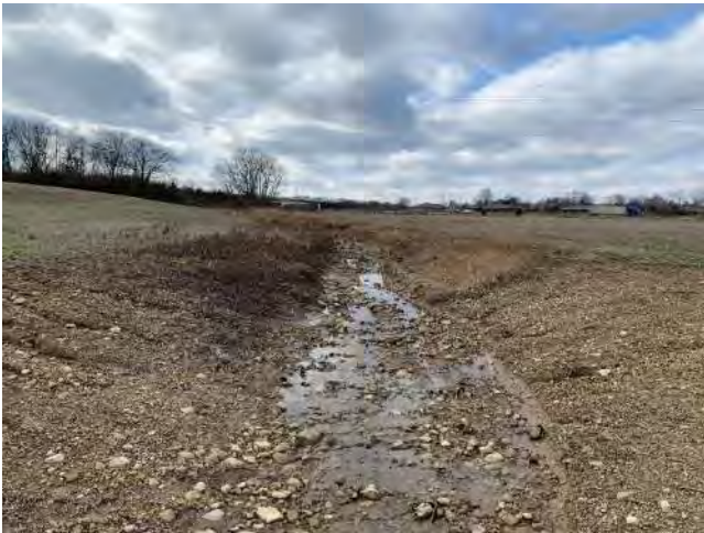
Stream ST-001, facing southwest – Jan. 2022
