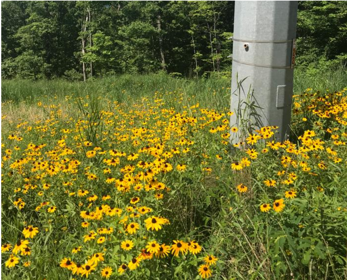
Figure 9. Proposed Seed Mix Planted Under Electrical Transmission Lines
