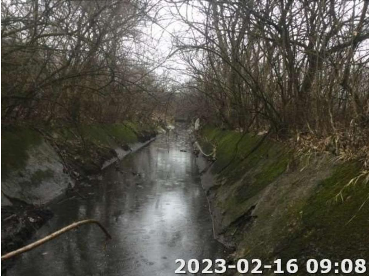
Figure 3. Current Ditch Condition (Facing West)
