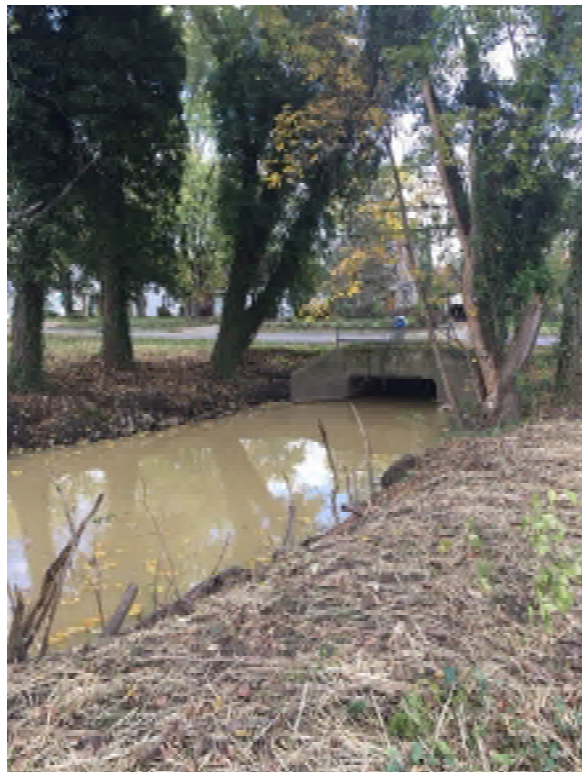
View of Bliss Run Culvert at E Livingstone Ave
