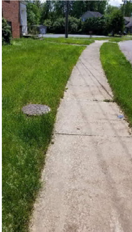
View of Sidewalk Along Brookwood Rd Facing South
