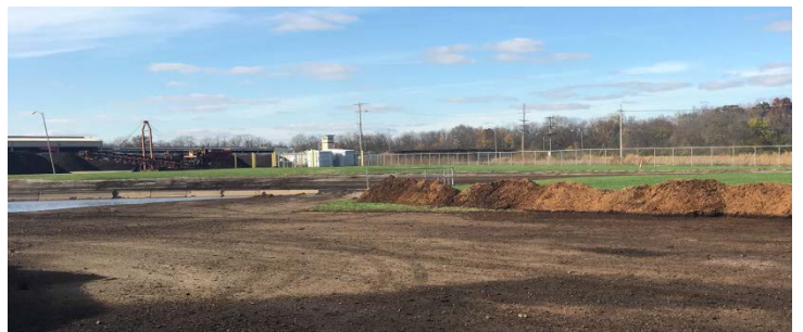
Partial view of the woodchip berm used to retain additional leachate during wet weather events.
