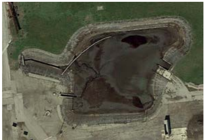
Compost Facility Leachate Lagoon is approximately 1.5 Million Gallons. The inlet channel is on the upper west (left) side. The outlets are intakes for two separate pump stations on the lower west side of the lagoon.
