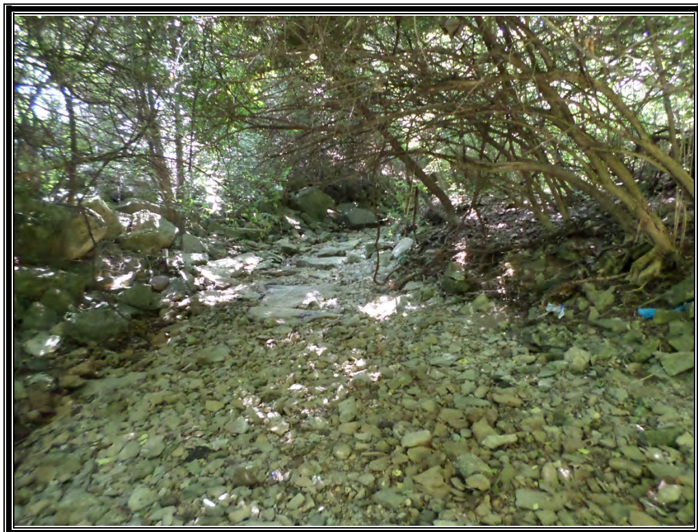
Photo 20 (6/14/16): Southeasterly view of the man-made drainage channel further down-gradient from the location of photos 16 through 19. Although perennial flow enters the property, this drainage channel does not carry surface water flow throughout. Flow enters unconsolidated material and becomes ground water.
