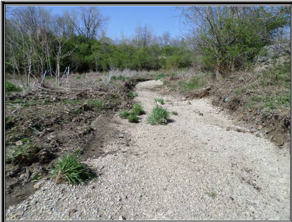
Photo 30 (4/20/16): Northeasterly view of the drainage channel on the southeast portion of the property.
