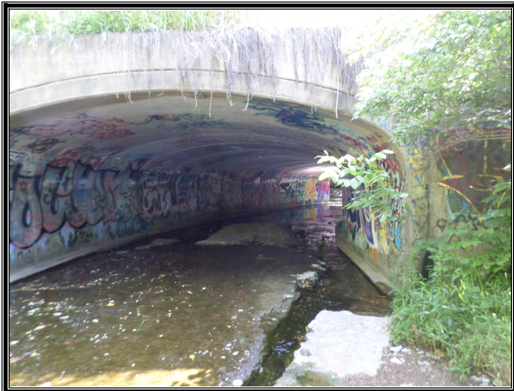
Photo 4 (6/14/16): Easterly view along Roberts Millikin Ditch and the culvert beneath Dublin Road. This photo is from off-site, west of Dublin Road.
