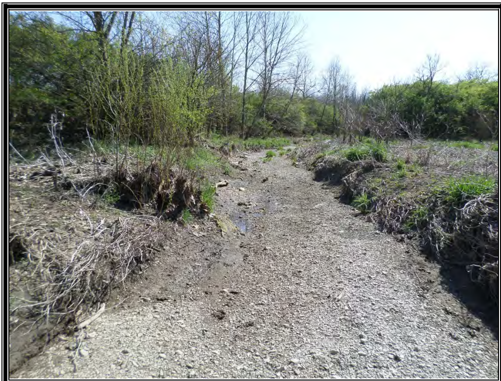
Photo 32 (4/20/16): Southwesterly view of the drainage channel on the southeast portion of the property.
