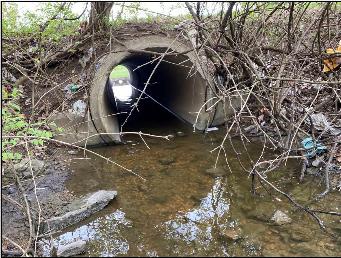
Photo 29 – Westerly view at the origination of Stream 9. This culvert pipe discharges surface water from a west adjoining storm water management pond.
