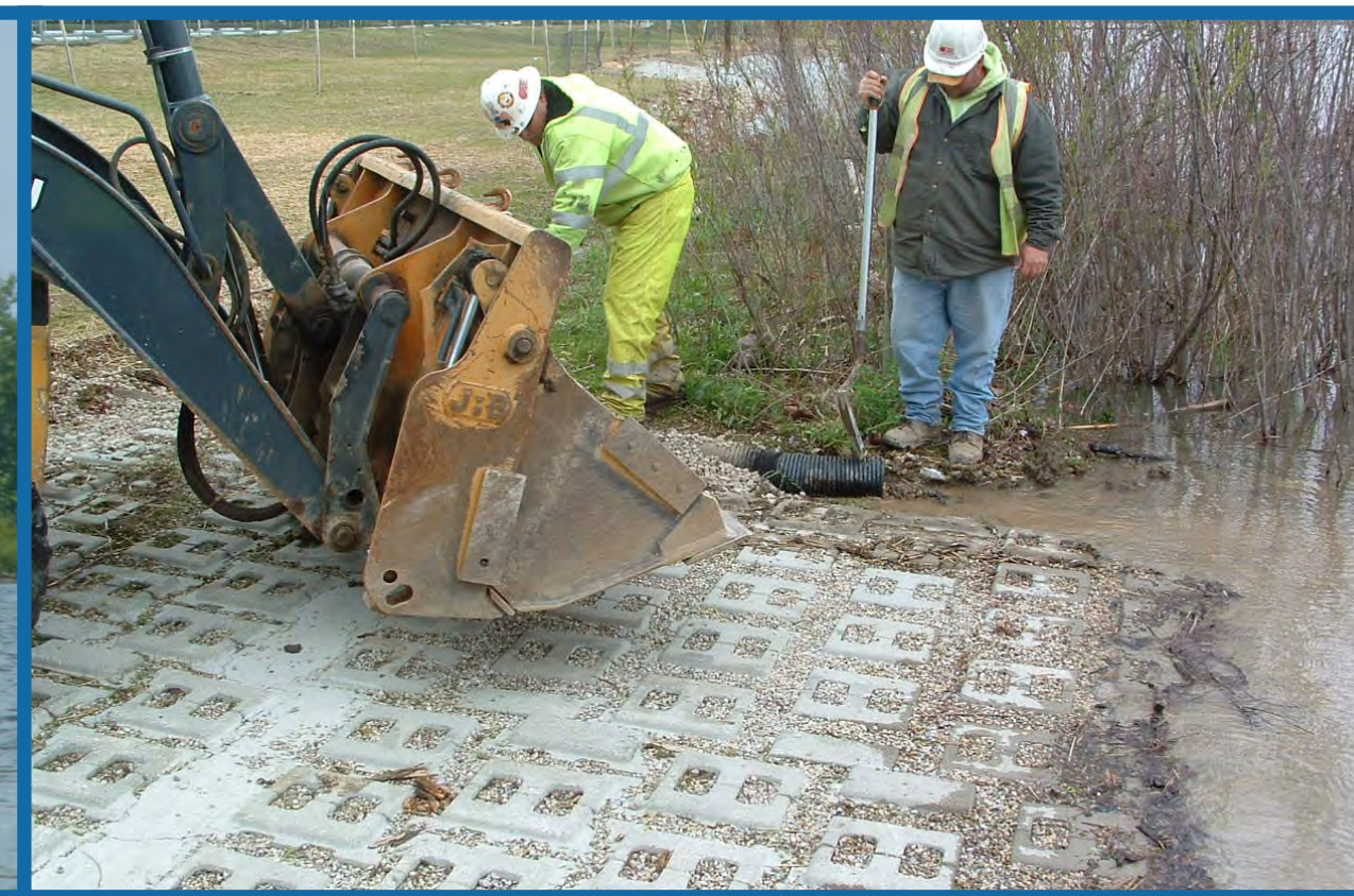
Armor-flex® holds soil and provides a hard, porous surface which can support grasses and foot traffic.
