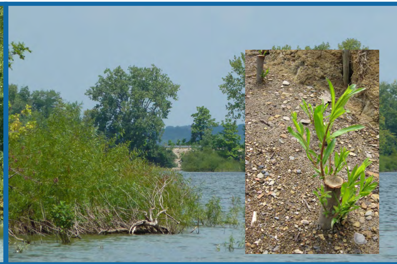
Live willow stakes will establish a fast growing, deep-rooted buffer at the water's edge.
