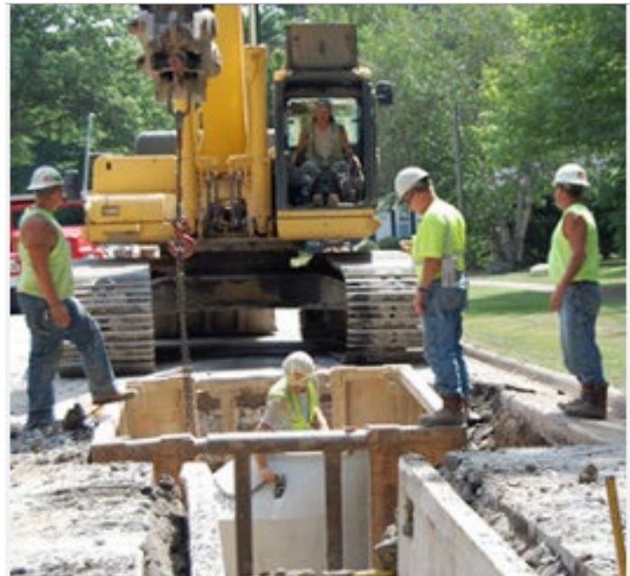
Installation of Sanitary Sewer
