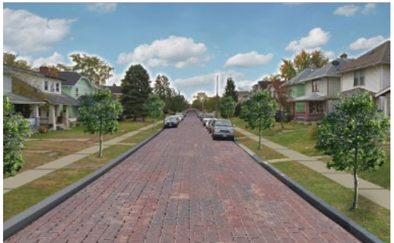
Permeable Pavers Installed on a Columbus Street
