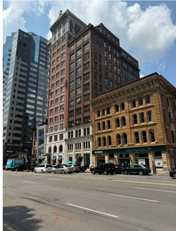
Broad Street Curbside Critical Access
