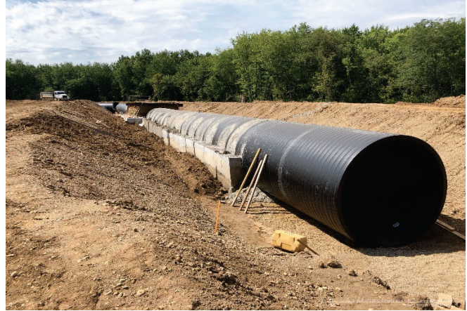
Photograph of the construction of the CEPT effluent pipeline at the Southerly Wastewater Treatment Plant.
