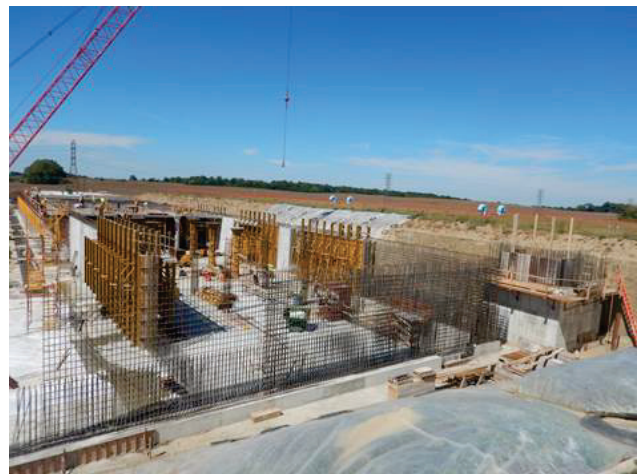
Installation of a new clearwell at PAWP. This will increase the reliability of the water supply system.
