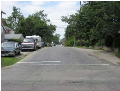
North/south street do not have sidewalks.
