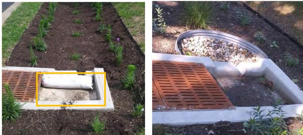
**Figure 4. Bioretention cell with sandbag blocking the inlet and the same cell after sandbag was removed and runoff from street was routed into the practice. Blocking of the inlet structures prevented high-intensity runoff events from entering the practice immediately following planting to allow juvenile plants to become established in the bioretention media. An additional erosion control practice downstream of the inlet weir was added after the sandbag was removed.**
